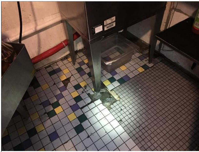
Photo 38: Minor cracking in floor tile behind bar area.
