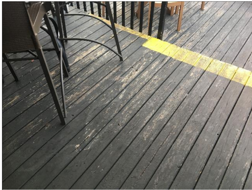
Photo 31: Typical wood decking with marked changes in elevation.
