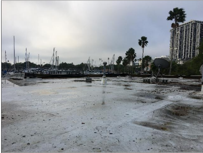
Photo 25: Typical TPO membrane installation at subject property.
