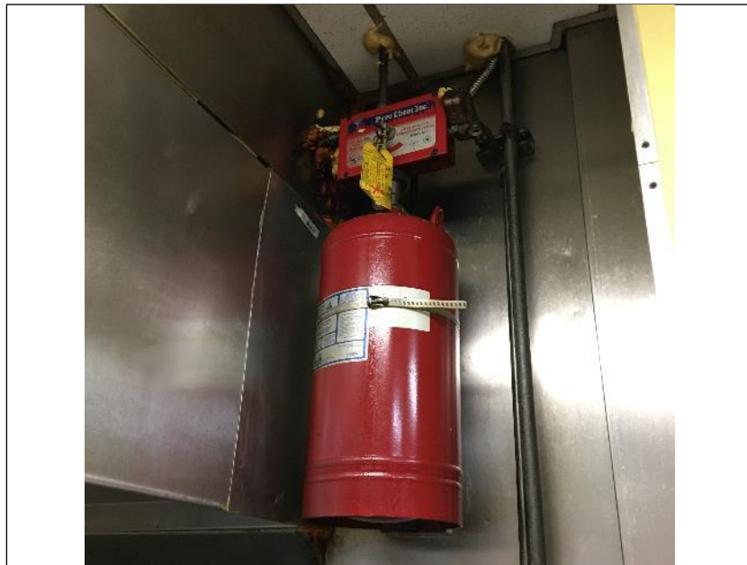
Photo 53: Automatic fire suppression system at kitchen grill.
