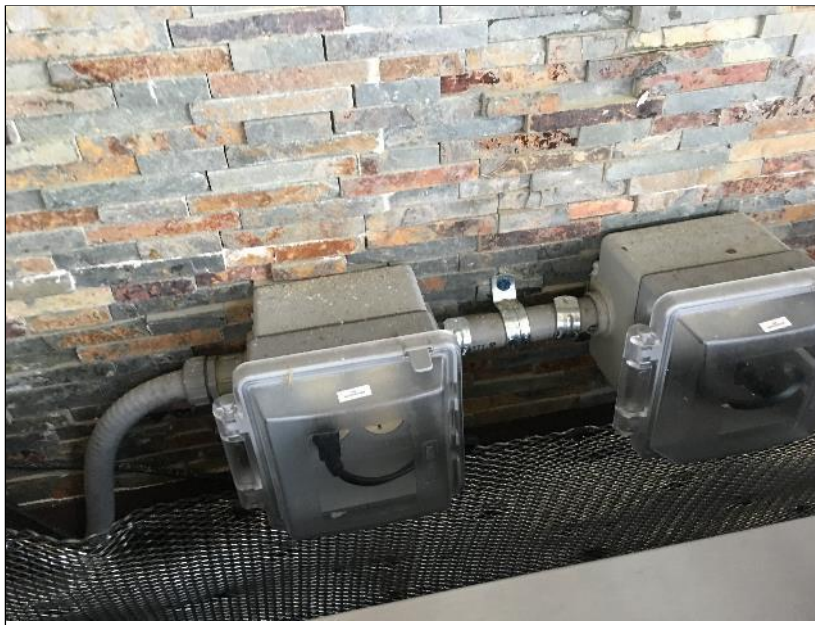
Photo 48: Weather protected exterior electrical outlets.
