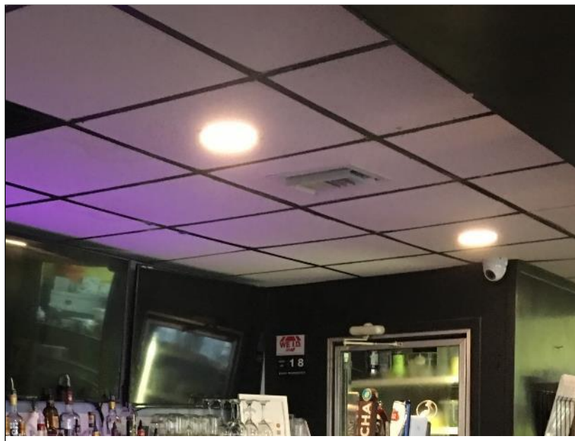
Photo 42: Air vents mounted on suspended ceiling.
