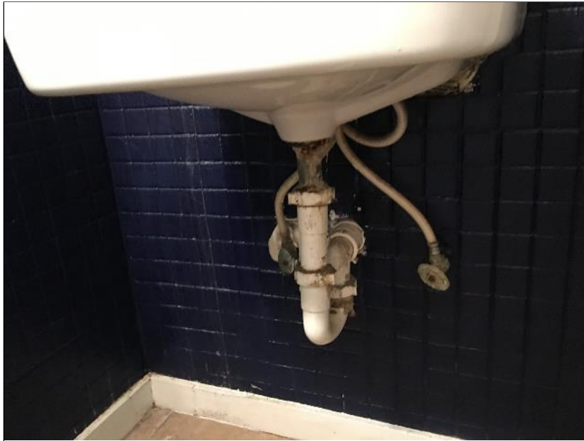
Photo 45: PVC drains at restrooms.
