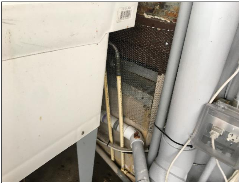
Photo 46: PVC plumbing behind outdoor bar.
