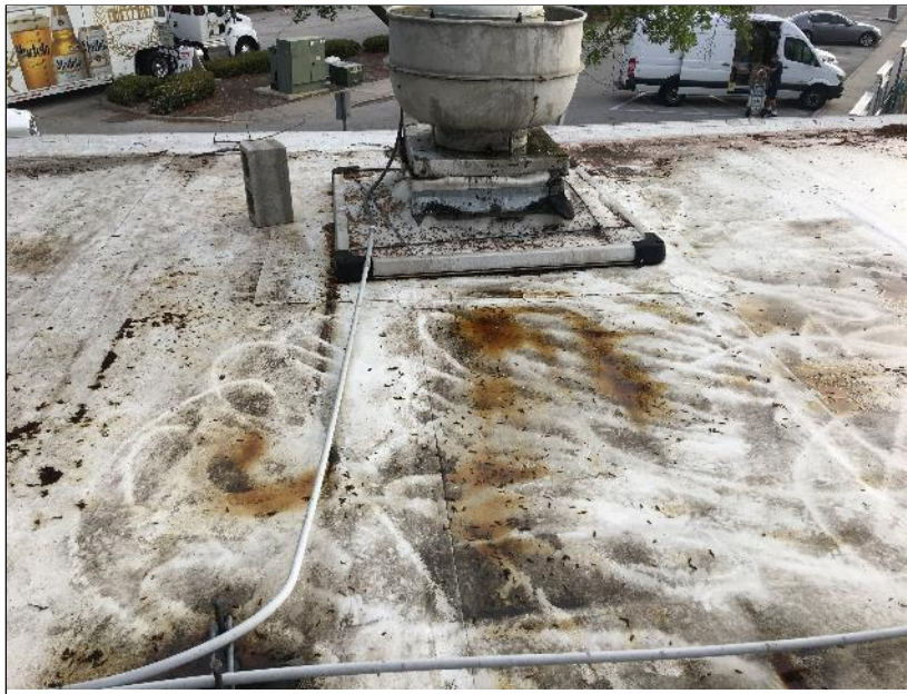
Photo 26: Observed grease residue near kitchen exhaust.
