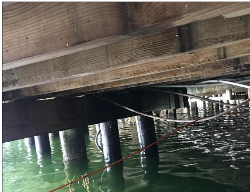
Photo 32: Typical wood decking supports and piles.
