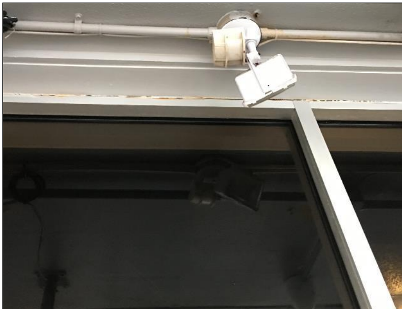
Photo 24: Detached sealant along header of storefronts.
